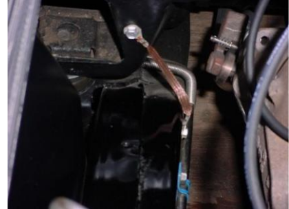
Fig 25. Connection of a ground strap to a chassis ground bolt. 29
