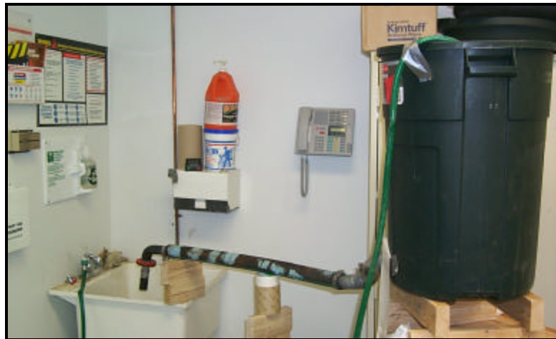
Figure 66: Horizontal filler tube with reducer elbow and check valve.
