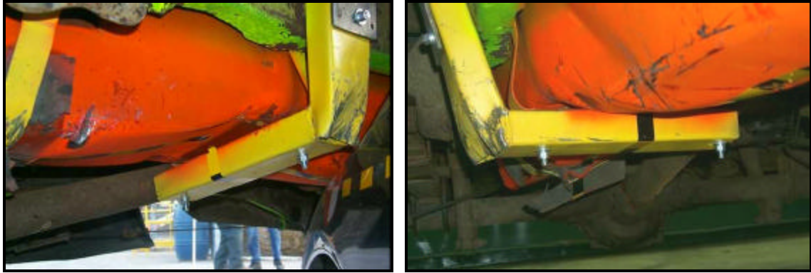
Figure 58: Deformations of the centre portion of the tank (test RP 01-039).
