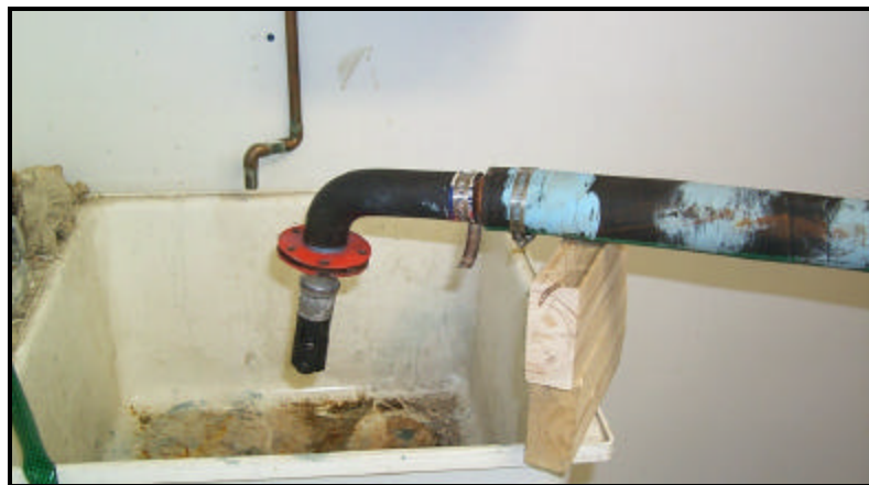
Figure 66: Horizontal filler tube with reducer elbow and check valve.
