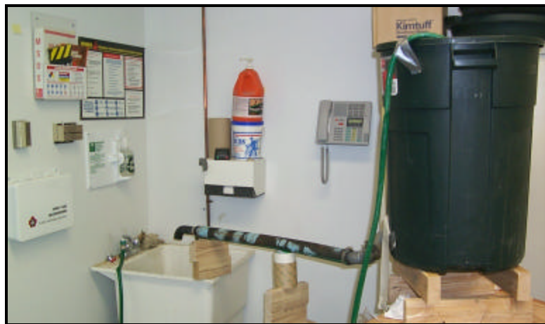
Figure 69: Horizontal filler tube with reducer elbow (NO check valve).
