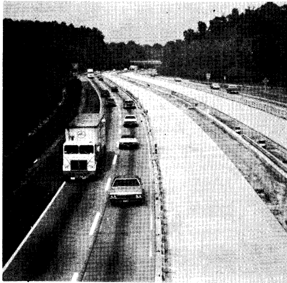
Figure 18. Timber barricades placed on edge of existing roadway adjacent to the median during construction stage one. Source: NTSB.
