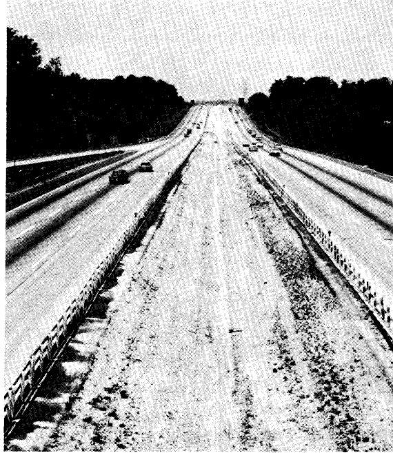
Figure 21. Timber barricades on a section of I-495 where for long periods of time no substantive work was being performed. Source: NTSB.
