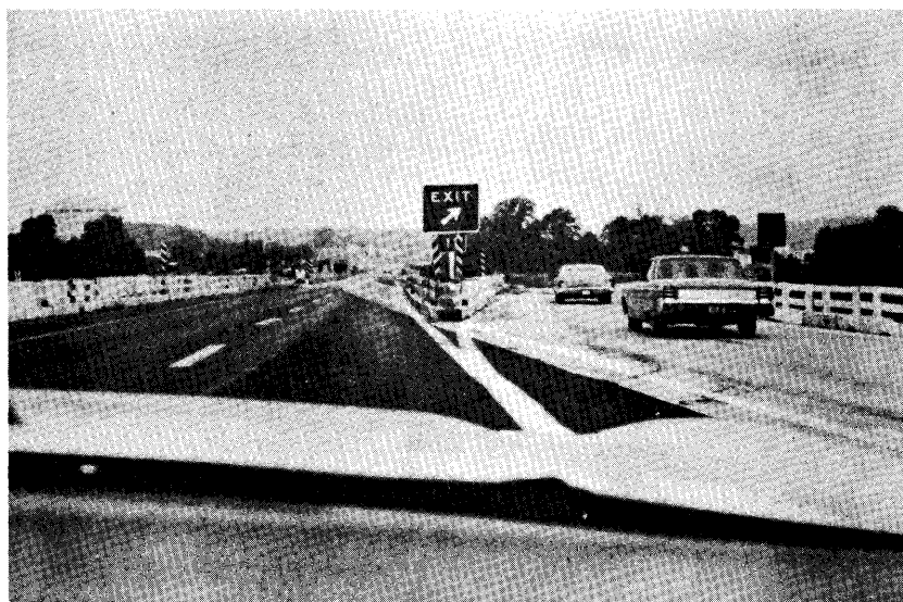
Figure 20. Timber barricades used for channelization at Exit 11 on I-495. Source: NTSB.
